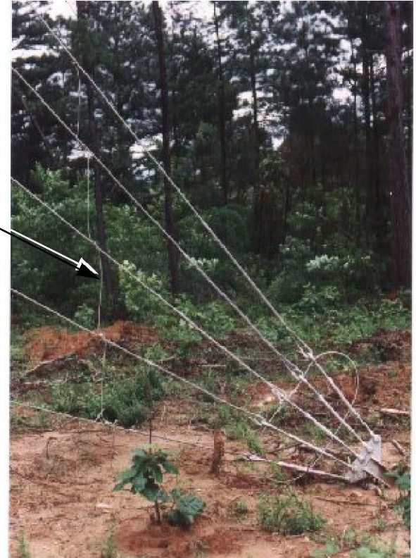
FIGURE 6-24 EXAMPLE OF TOWER GUY WIRE GROUNDING
