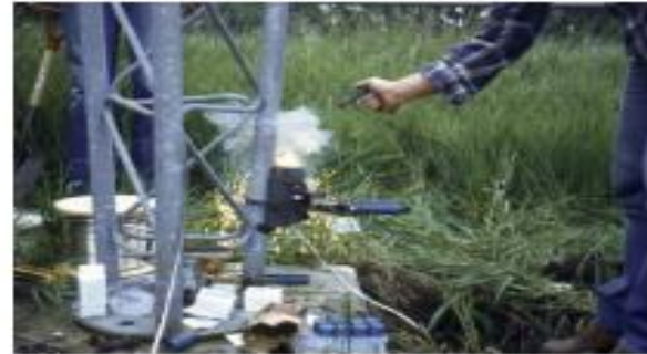
FIGURE 6-48 EXOTHERMIC WELDING MOLD (LEFT) AND PROCESS (RIGHT)
