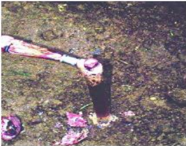
FIGURE 6-49 COMPLETED EXOTHERMIC WELDS IN TRENCH AND ON TOWER
