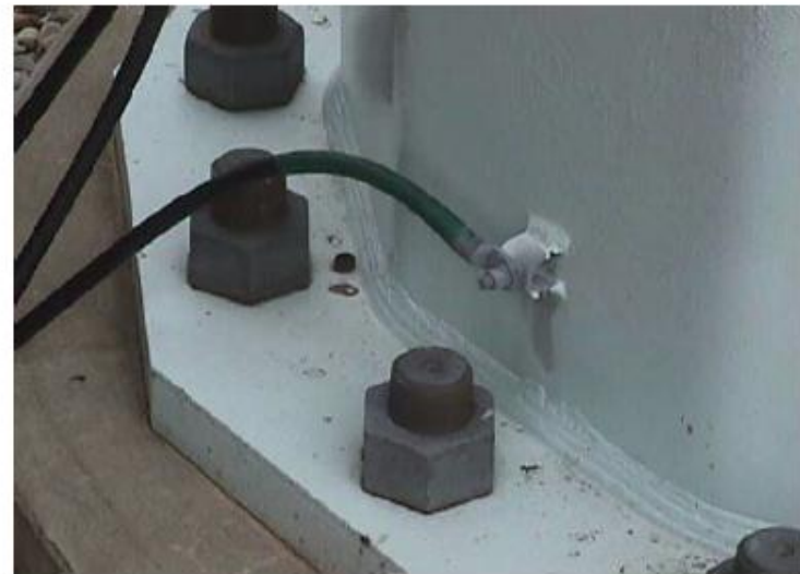
FIGURE 6-26 EXAMPLE OF MONOPOLE TOWER GROUND CONDUCTOR
