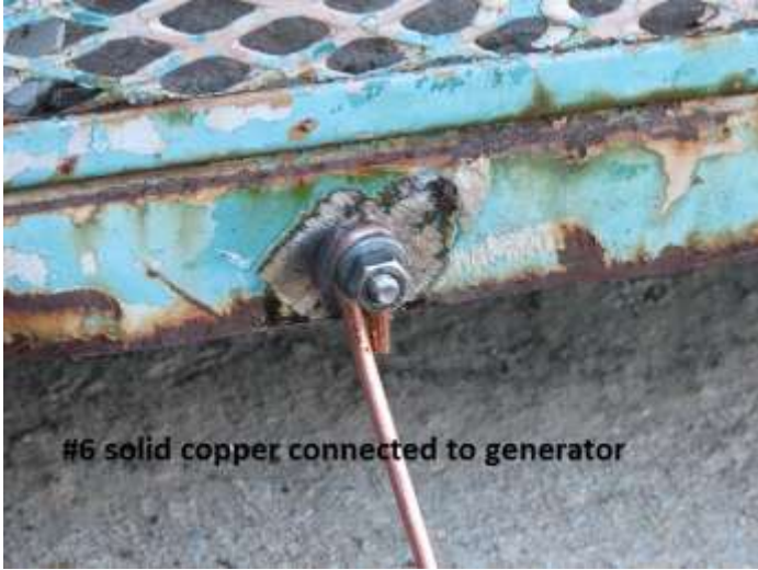
Copper ground strap under bench
